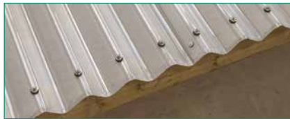
1 Primary Fixing at every corrugation
